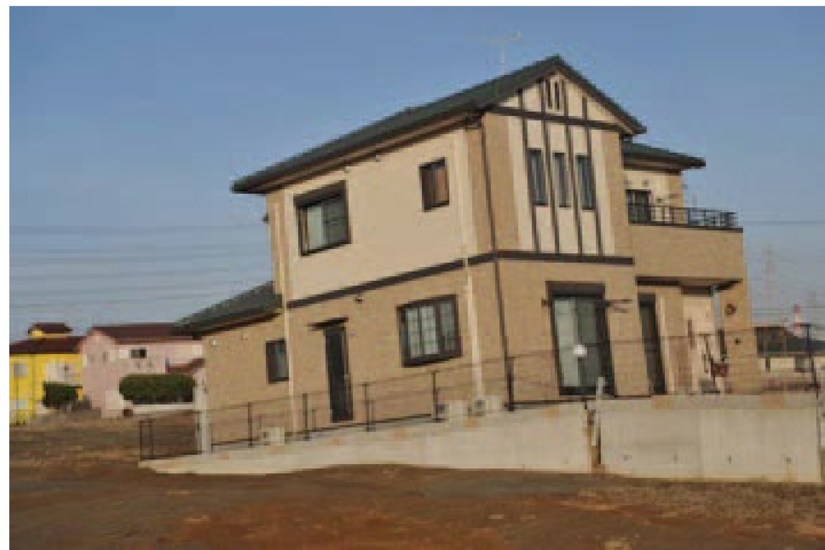
Tilted damage caused by liquefaction in Tohoku earthquake (Tokimatsu et al., 2012)
