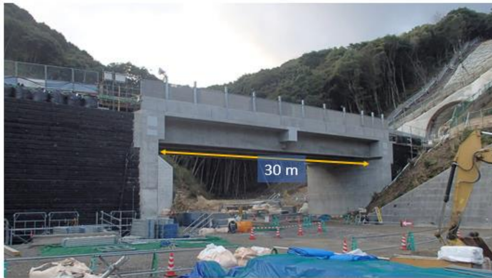
GRS Integral Bridge at Genshu for Kyushu Shinkansen, 2018
